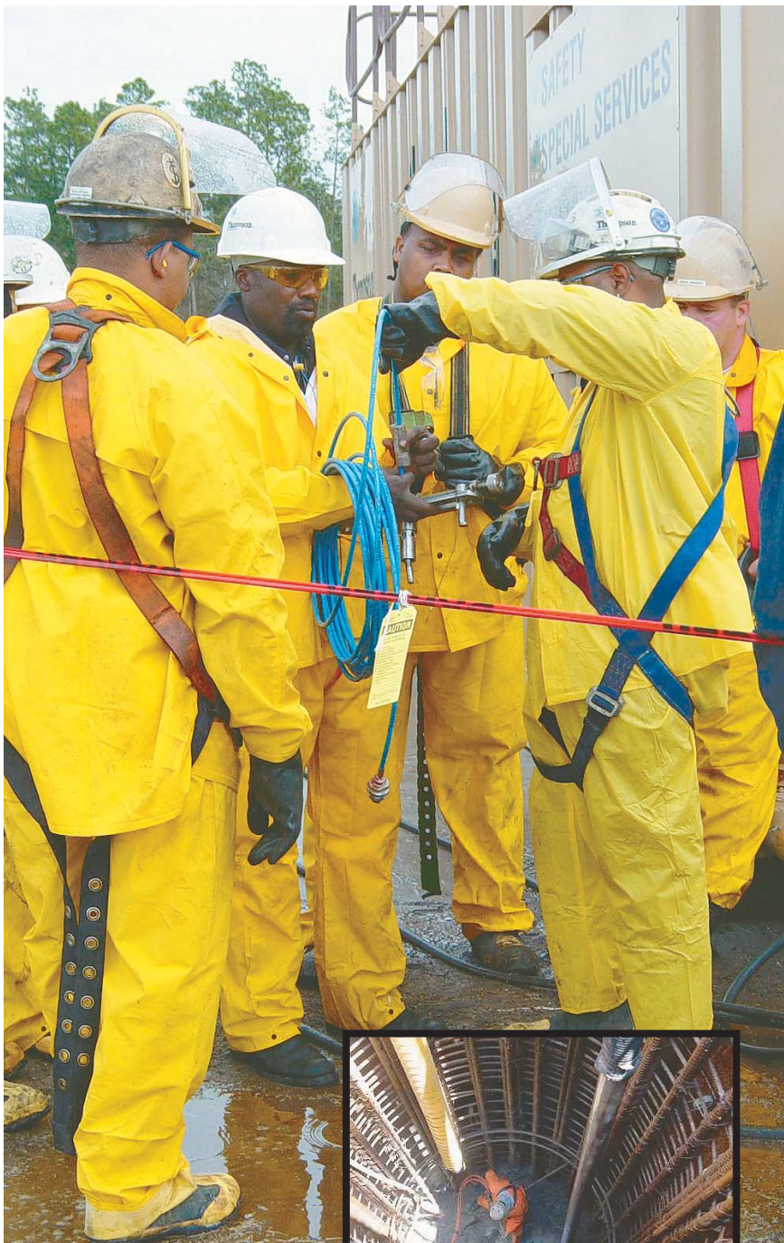
Above: Eric Miller, technical skills instructor with Thompson Industrial Services, shows a group of trainees how to use one of the required water blaster safety devices. Right photo: Technicians use water blasting to prepare a bridge caisson for the new Cooper River bridge in Charleston, S.C.
