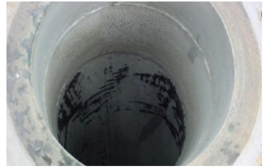
Before sponge blasting & after chemical cleaning
