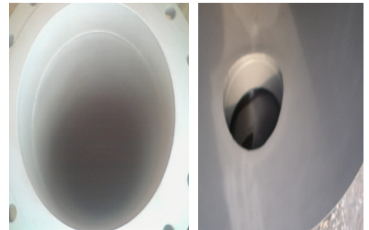
After sponge blasting – achieved the maximum degree of cleaning
