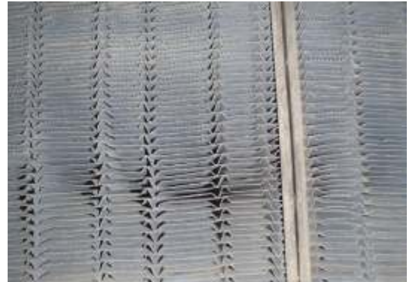
Properly Cleaned Catalyst Providing Maximum Surface Area
